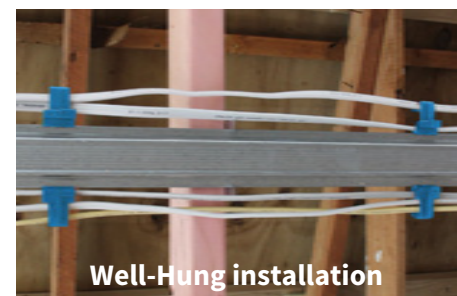
Typical cable installation
